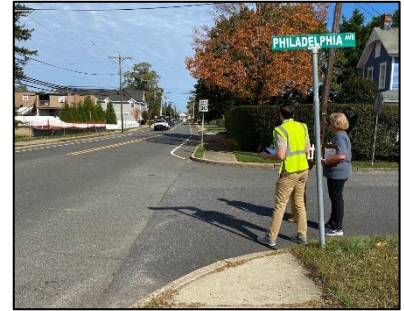
Picture 9: Intersection missing curb ramps on Arnold Avenue
