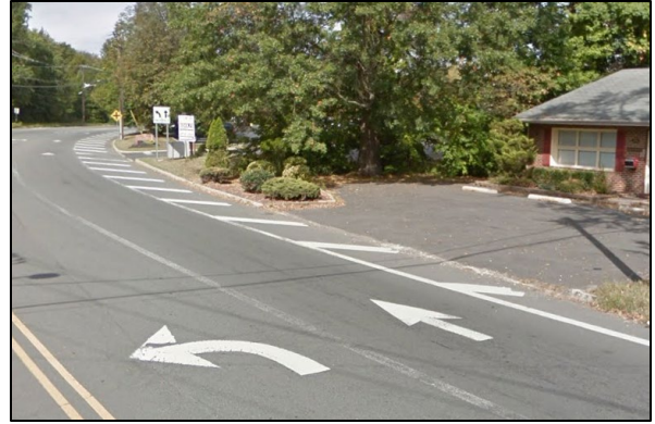
Picture 20: Example of striping used to narrow a lane on Young Road in Hamilton Township.
