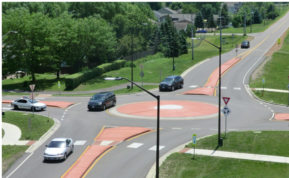
Example of a single-lane roundabout. Source: FHWA
