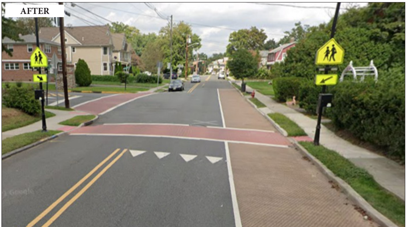
Figure 4 - After (2019) the raised intersection in Town A. (Source - Google Street View)
