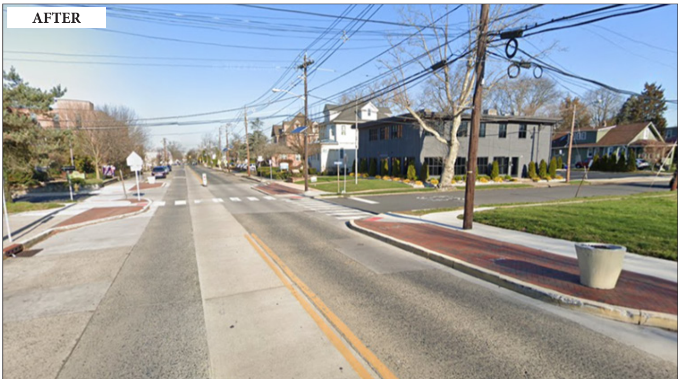
AFTER Figure 6 - After (2022) curb extensions in Town B. (Source: Google Street View)
