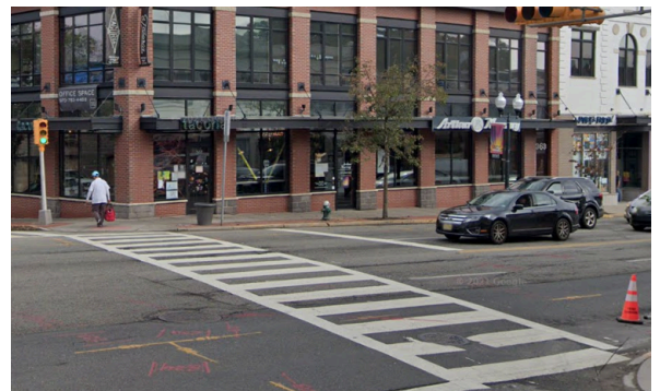
High-visibility crosswalk with a cone on the street to warn of a pothole.
