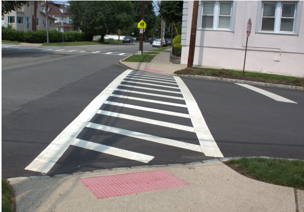
High-visibility crosswalk with truncated dome pads crossing Elmwood Ave.
