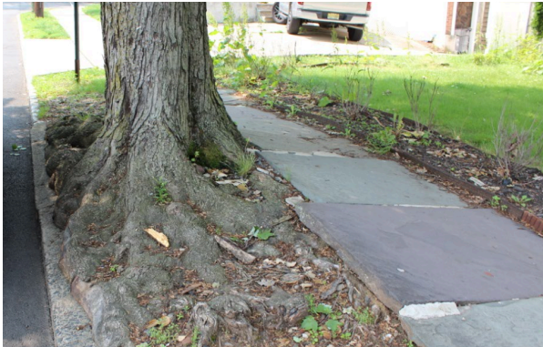
Sidewalk is elevated due to tree roots.
