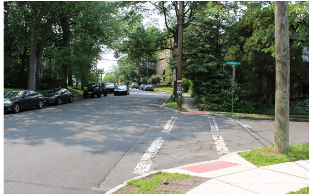
Truncated dome pad and faded crosswalk.
