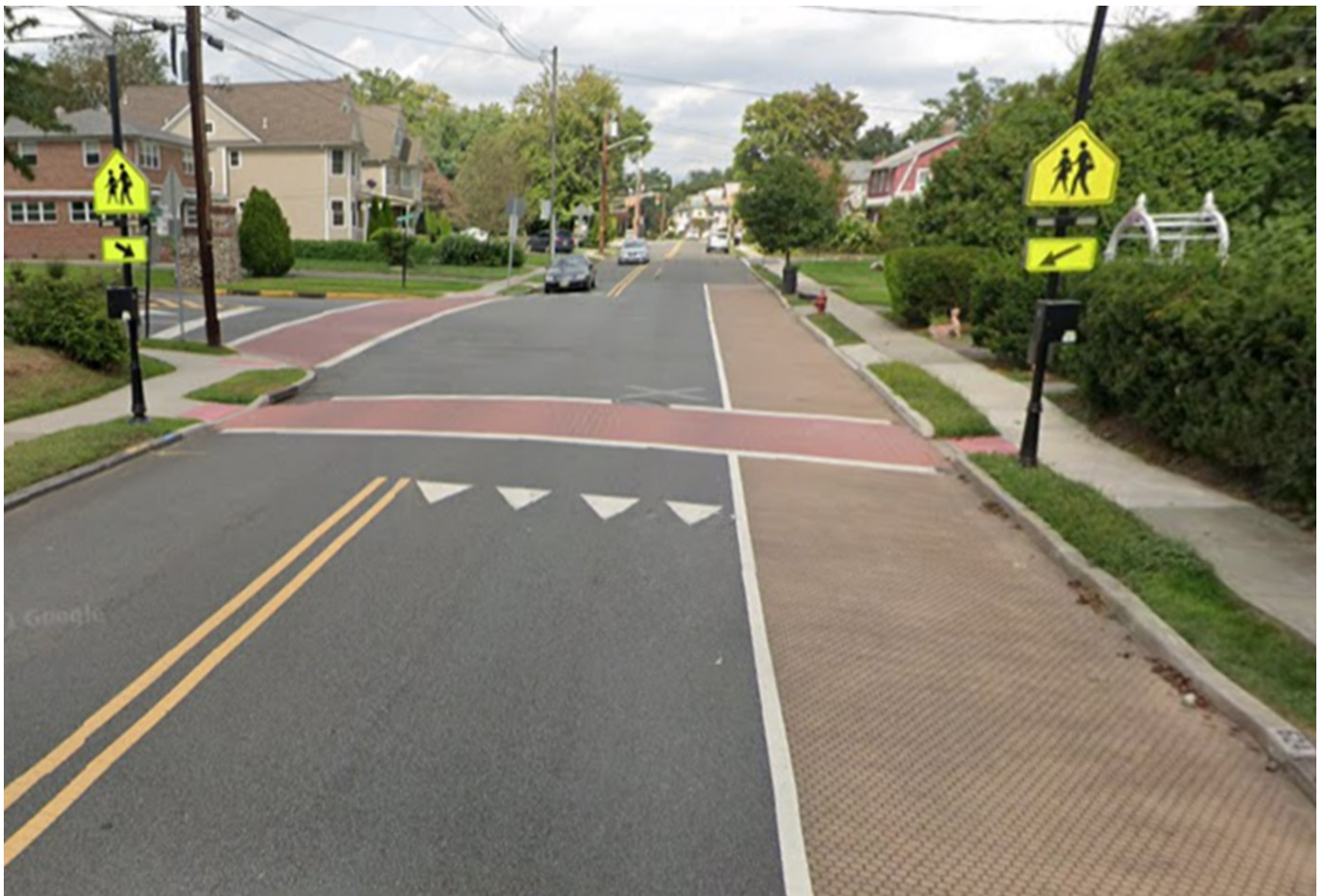
Figure 2: Case Study 1 after the treatment was implemented (2019)
