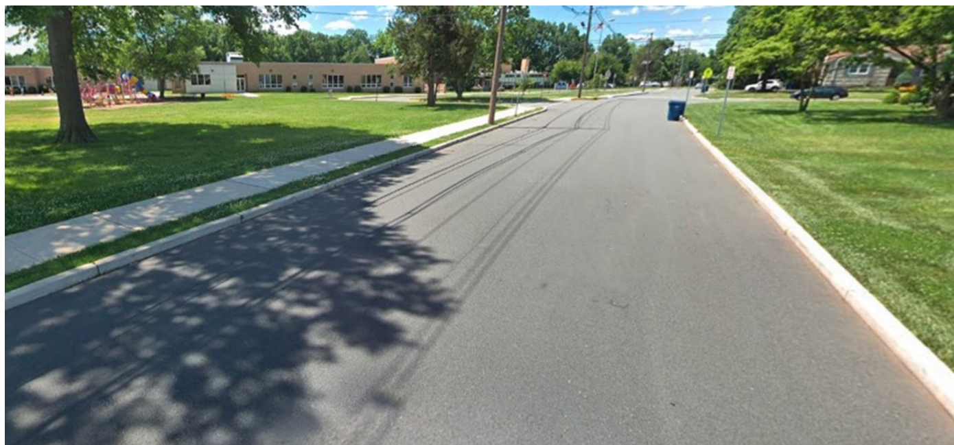
Figure 6: Case Study 3 after the treatment was implemented (2018)
