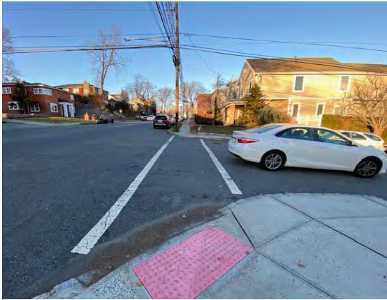
Misaligned dome pad
