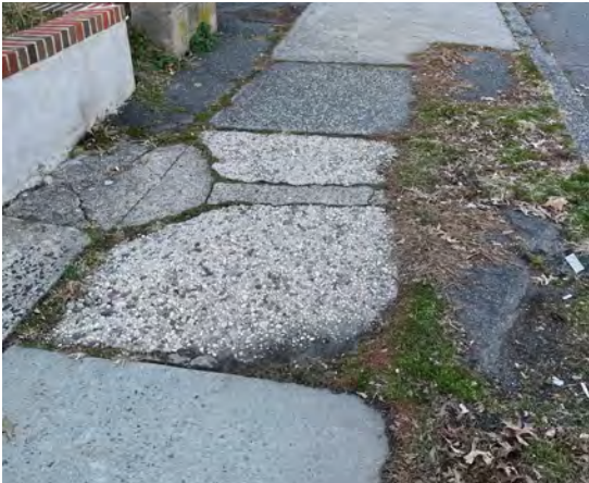
Cracked sidewalk
