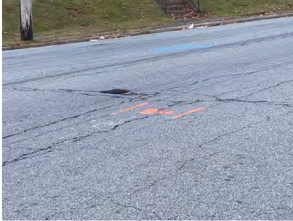
Pothole & cracks
