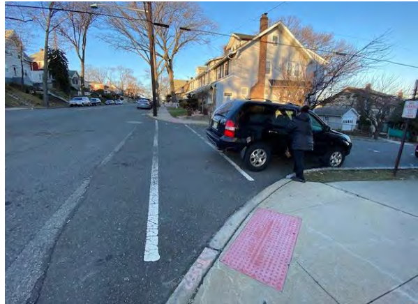
Low visibility crosswalk, wide turn radius
