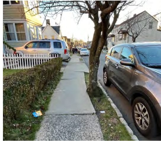
Uneven sidewalk & low hanging branches
