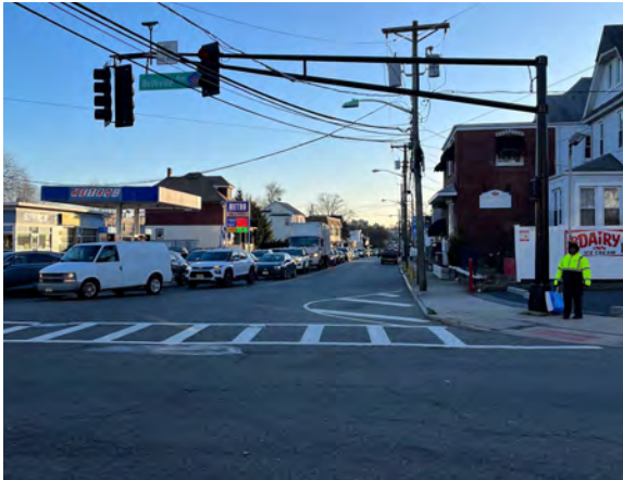
Small painted bump out present on the right to discourage parking
