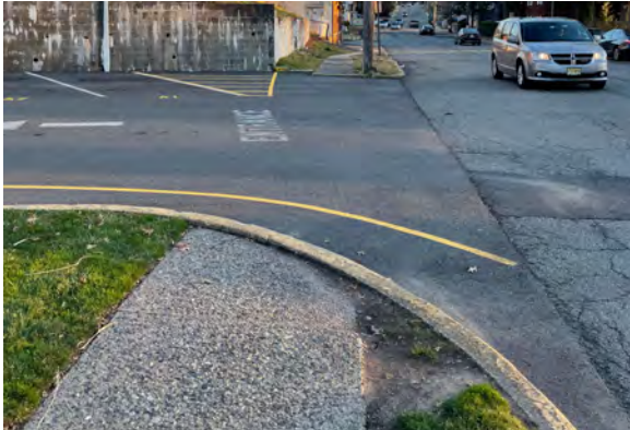
No crosswalk or truncated dome pads
