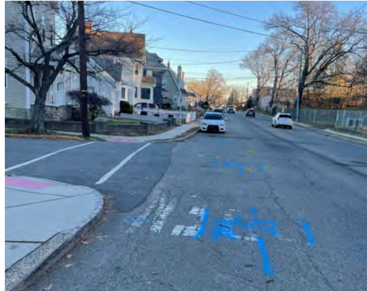
No stripes in crosswalk
