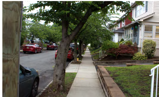
Sidewalk in good condition
