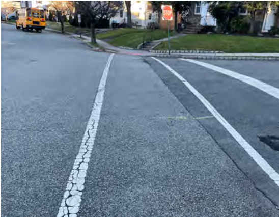
No stripes in crosswalk
