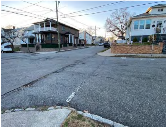
Fade crosswalk, no dome pads
