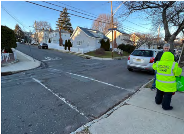
Faded low visibility crosswalk
