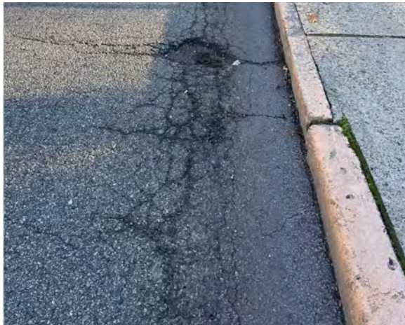
Pothole & cracks
