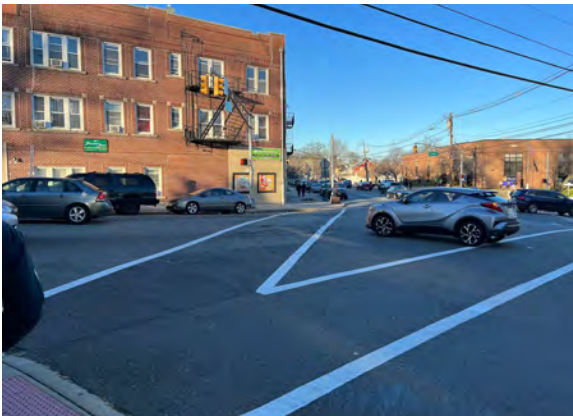
No stripes in crosswalk
