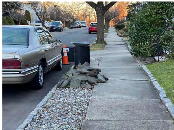
Rocks and raised sidewalk are trip hazards
