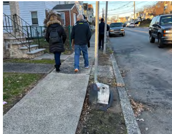
Litter/debris by pole
