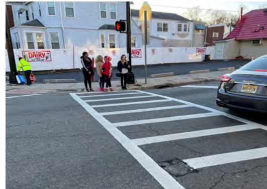
Pedestrian signal heads & high visibility crosswalk
