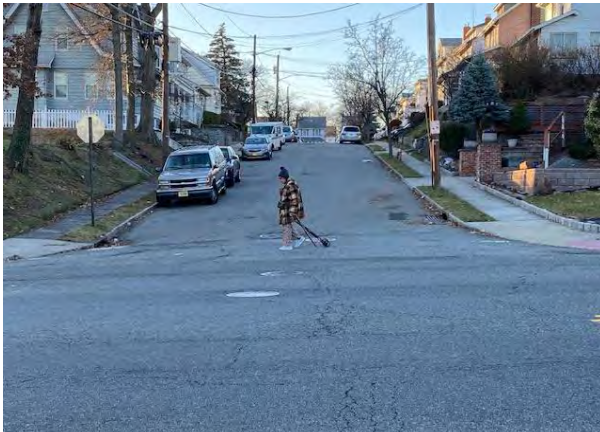
Crosswalk paint is faded/missing
