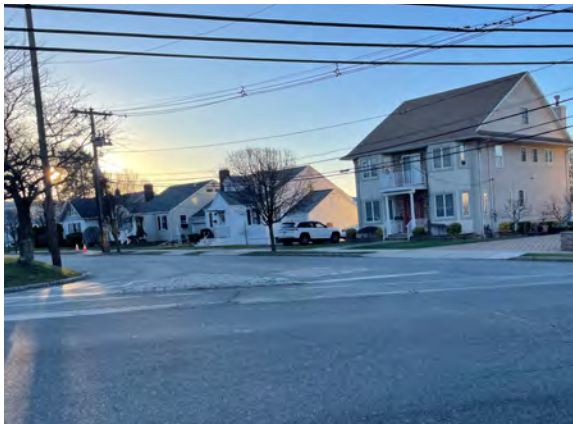
Long, faded crosswalk
