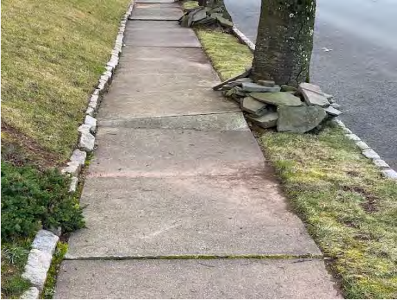
The sidewalk is uneven
