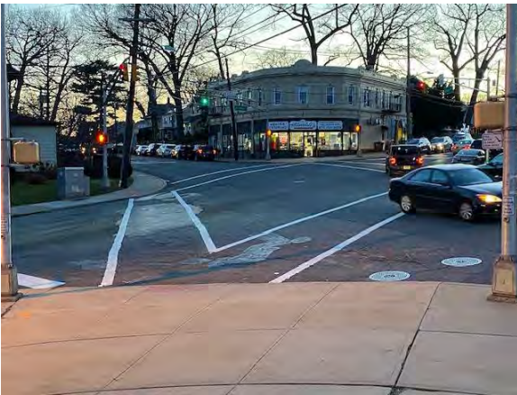
Lack of lighting at left corner
