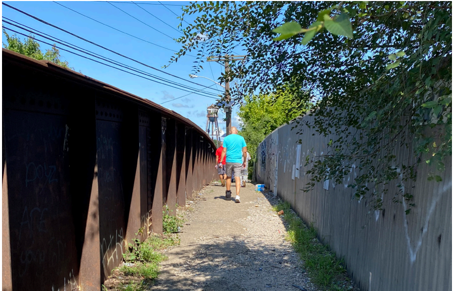
Figure 32 - Pedestrian walkway on the N. Olden Ave Bridge over the train tracks
