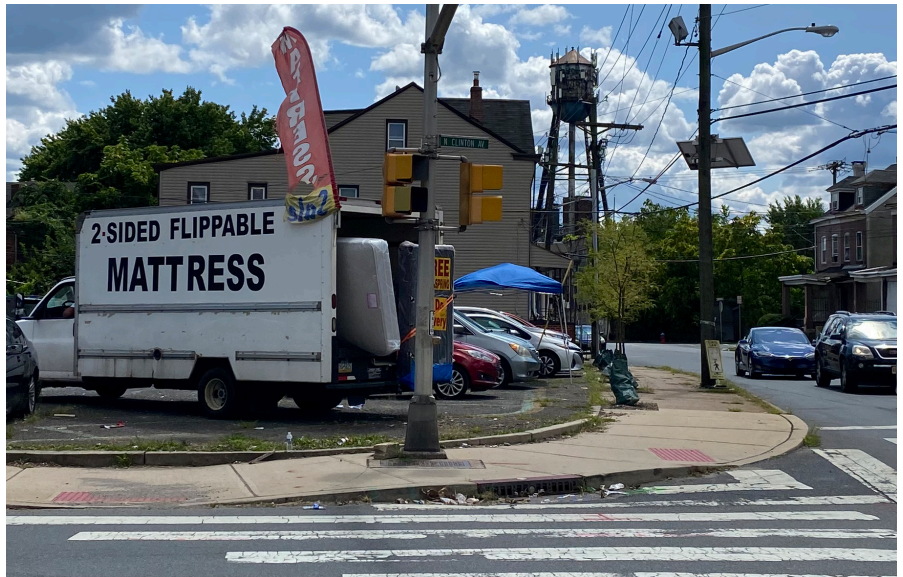
Figure 37 - Misaligned pedestrian signals at N. Clinton Ave & N. Olden Ave
