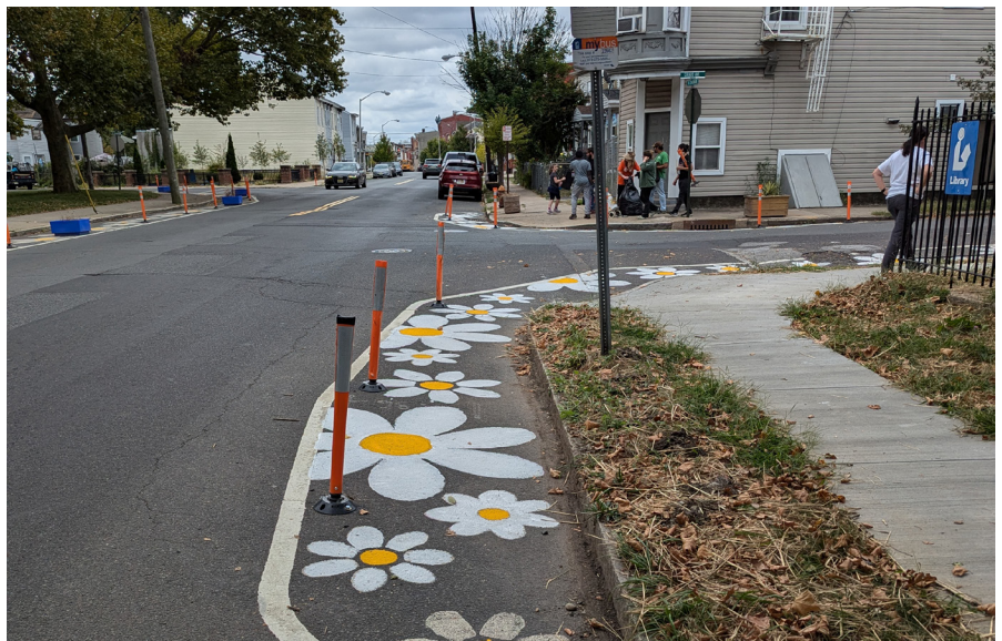
Figure 44 - Quick-build daylighting at Girard Ave and N. Clinton Ave intersection
