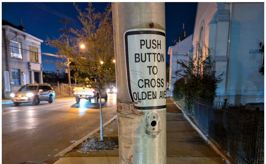
Figure 38 - Pedestrian push button missing from signal pole after being hit by a vehicle
