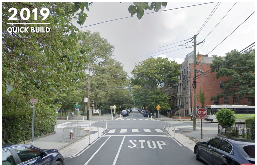
Figure 28 - Intersection with quick-build curb extensions using flex posts and paint
