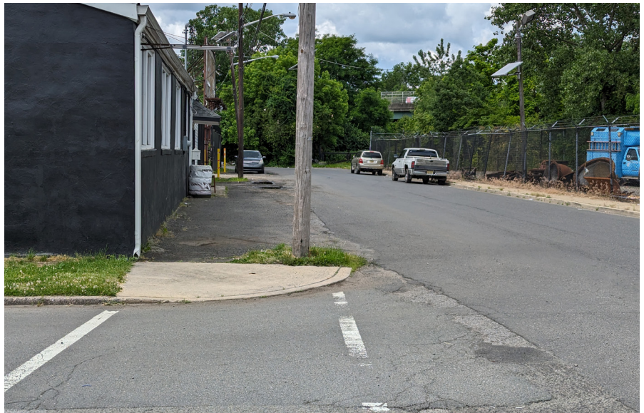
Figure 42 - Missing Sidewalk on Cortland St. Between Sherman Ave & Houghton Ave
