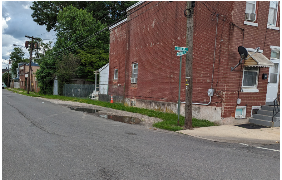
Figure 43 - Missing sidewalk on Courtland St. at Girard Ave
