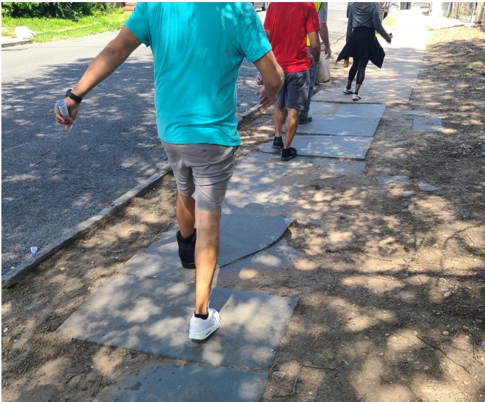
Figure 15 - Slate sidewalk in poor condition on Girard Ave
