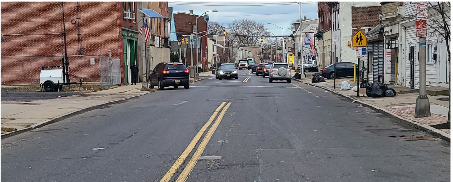
Figure 23 - Wide lanes on N. Clinton Ave
