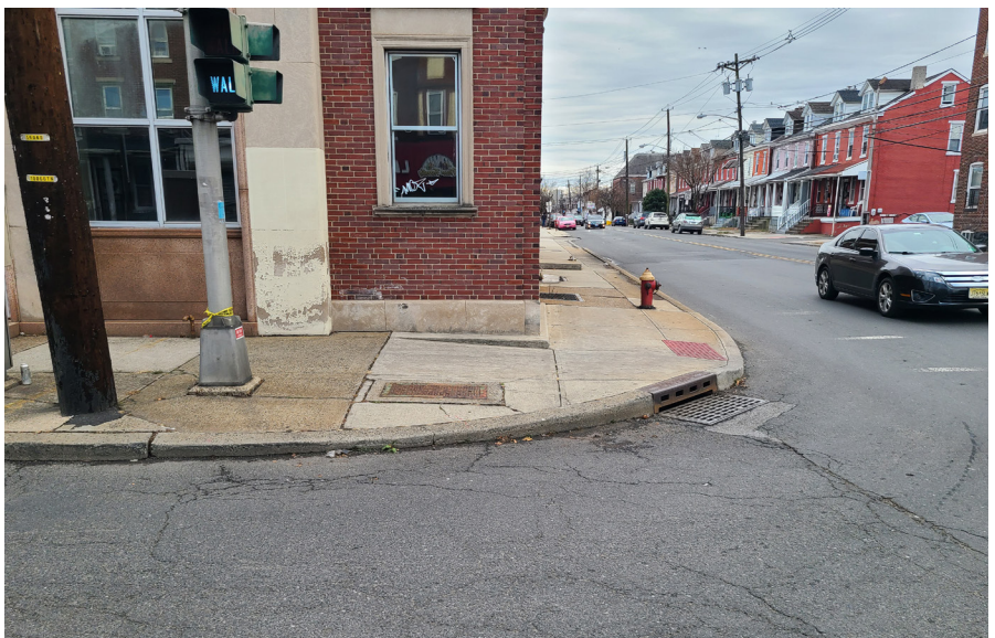
Figure 41 - No curb cuts at the northwest corner of E State Street and N Olden Ave
