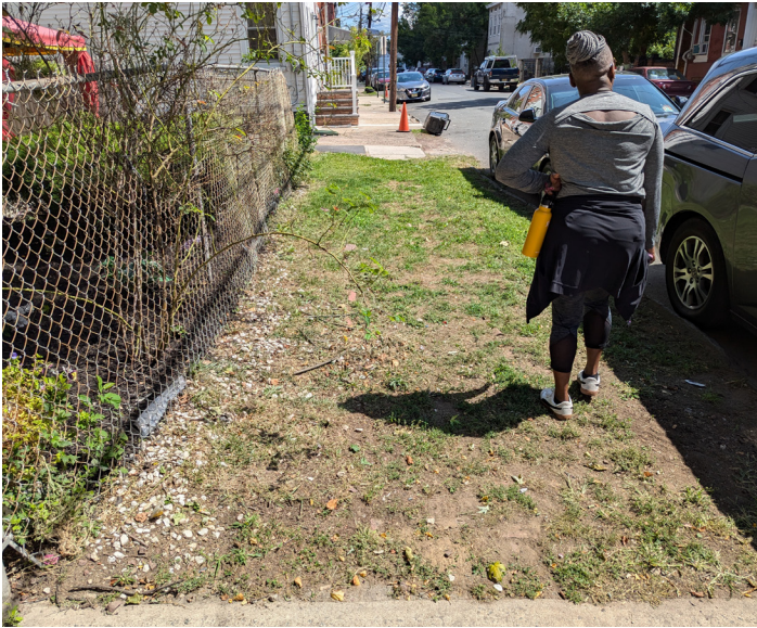
Figure 13 - Missing sidewalk on Klagg Ave near Girard Ave
