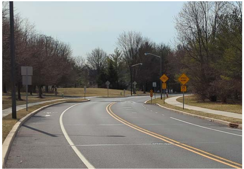
Figure 20 - Bike lanes, curb extension and raised crosswalk on Denow Rd
