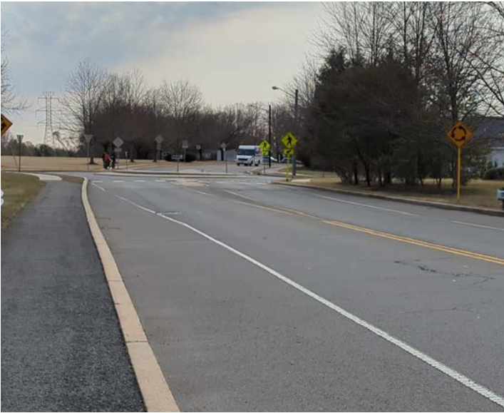
Figure 23 - Western approach to Denow roundabout
