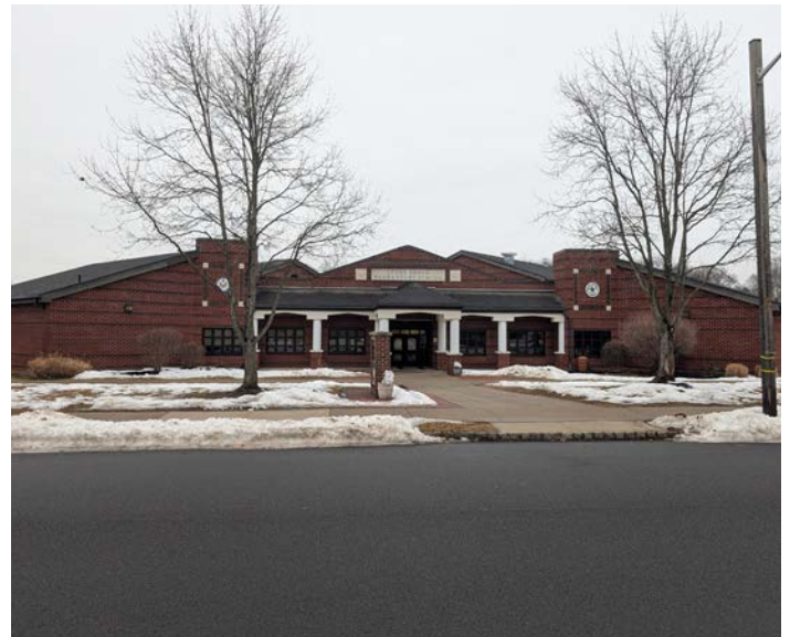
Figure 11 - Front of Stony Brook Elementary School
