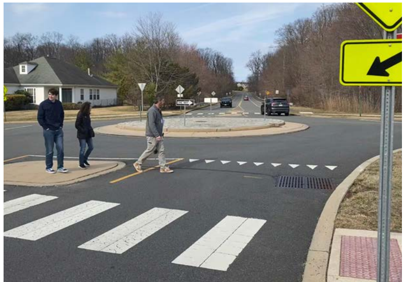
Figure 21 - Crosswalk too close to yield line at Denow Rd Roundabout
