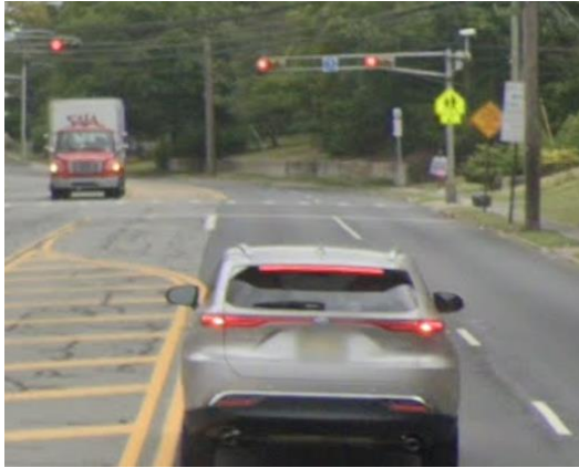
Left turn lane removes shoulder for cyclists Consider one thru lane & shoulder/bike lane
