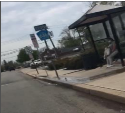
Good bus shelter
