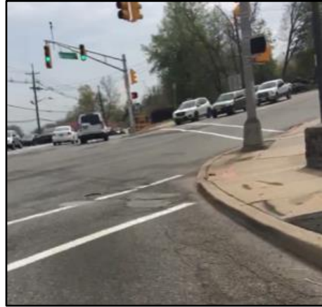
Long crossing distance and no stripes in crosswalk
