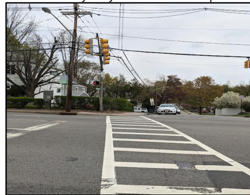
High visibility crosswalk, but long distance to cross
