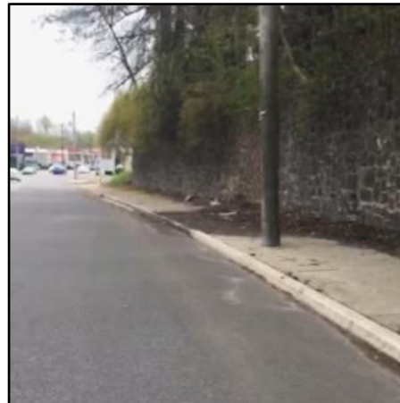
Debris and water building up on sidewalk
