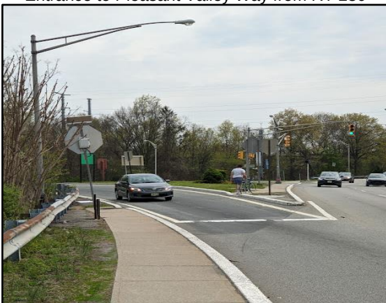
Sidewalk curb ramp is behind stop sign/bar. Repaint stop bar and STOP pavement marking and reposition stop sign so cars stop in front of a painted crosswalk.
