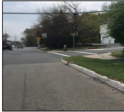
No strips in crosswalk
