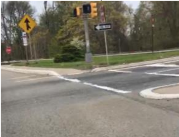
Low visibility crosswalk. The median curb is slightly raised higher than the street.
