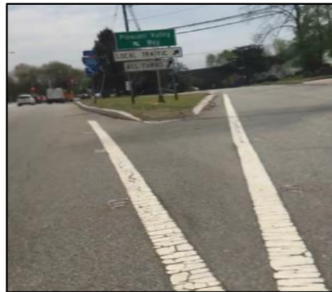
No crosswalk to access Bus stop on median
