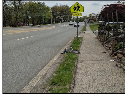
Sidewalk is very close to street, no shoulder
