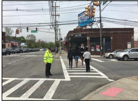
High-visibility crosswalk with pedestrian signal and crossing guard. Lacks lighting and dome pad is directed toward the intersection.
