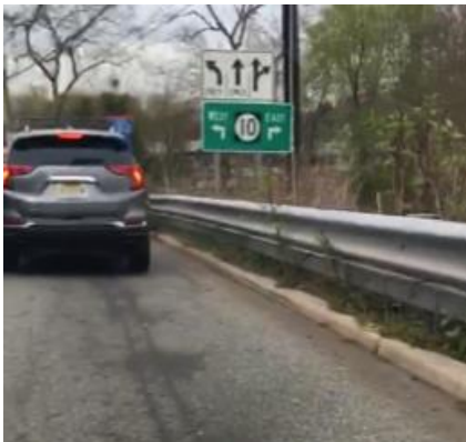
Road widens approaching Intersection with Mt. Pleasant Ave. No sidewalk available.
