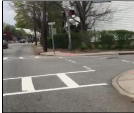
No stripes in crosswalk across Hooper Ave
