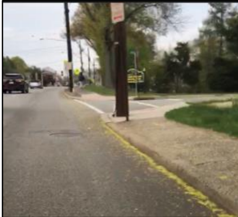
Utility pole obstructs sidewalk
