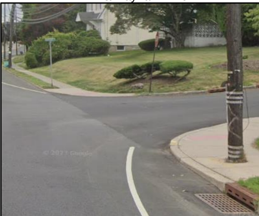
Need high-visibility crosswalk
