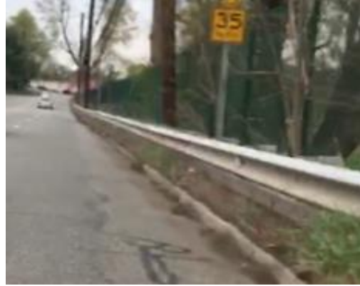
No sidewalk on northbound side
