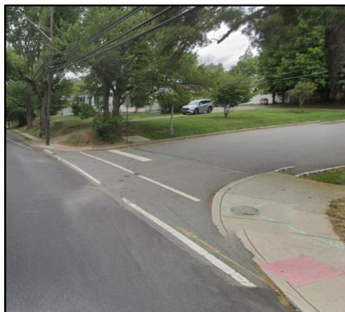
Need high-visibility crosswalk
