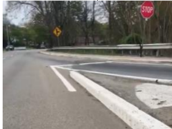
Crosswalk is placed 10 feet before the stop sign and stop bar, meaning pedestrians cross before cars stop. Suggest moving crosswalk in front so stopped cars will see pedestrians cross - add lights/Ped Crossing Sign.
