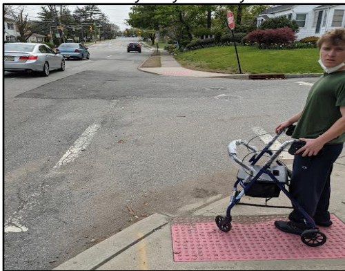
Dome pad aligned correctly, no stripes in crosswalk
